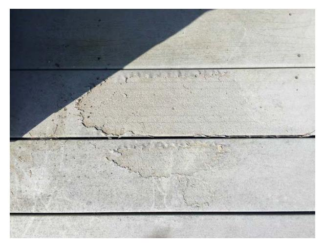
470. The following photograph is a true and accurate representation of the cracking Giovannetti's Decking is experiencing as of September 24, 2015:
