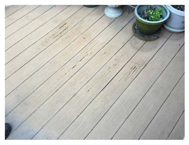
431. The crumbling has become so severe that the Decking is no longer safe to walk on and is in danger of collapsing.
