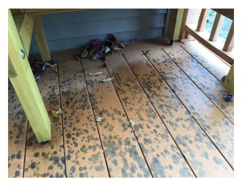
367. The following photograph is a true and accurate representation of the warping and mold growth Claxton's Decking is experiencing as of October 24, 2015:
