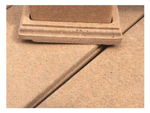
398. The following is a true and accurate representation of the mold growth Turcheck's Decking is experiencing as of August 24, 2015:
