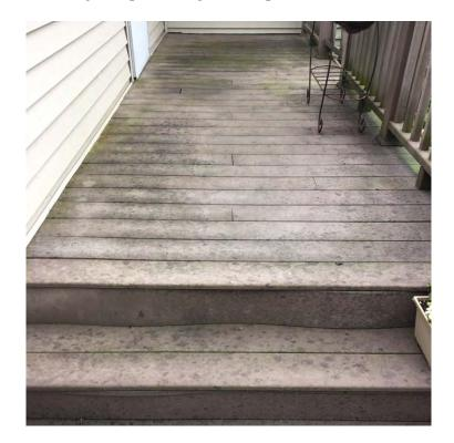
376. The following photograph is a true and accurate representation of the warping and mold growth Ernst's Decking is experiencing as of September 19, 2015:
