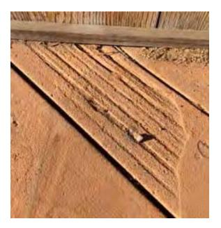
600. The following photograph is a true and accurate representation of the shrinking experiencing by Koster's Decking:
