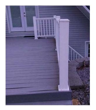
569. The following photograph is a true and accurate representation of the cracking and warping experienced by King's Decking as of March 18, 2015:
