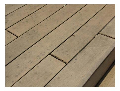
301. The following photograph is a true and accurate representation of the shrinking and fading experienced by Sheridan's Decking as of August 20, 2014:
