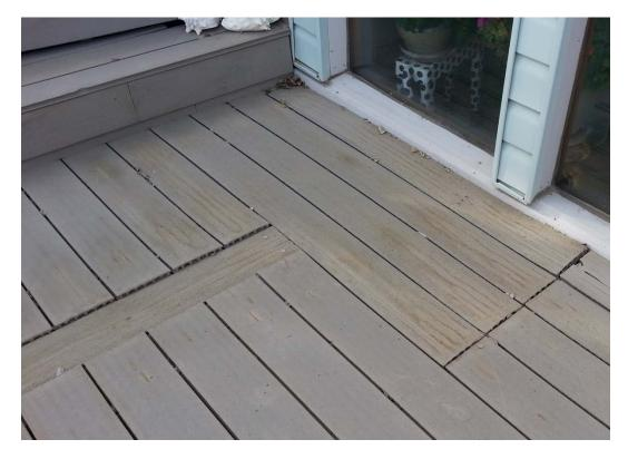
410. The following photograph is a true and accurate representation of the cracking and crumbling Tuthill's Decking is experiencing as of March 14, 2015:
